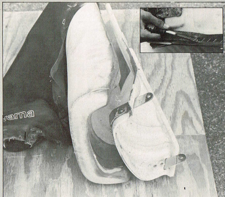
The first step is to remove your old cover. Use a slot screwdriver and pop out all of the staples.
