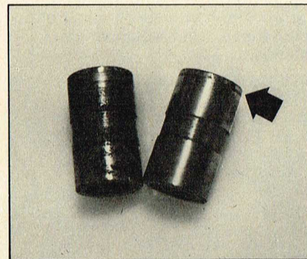
When replacing the bushing/bearing it's usually a good idea to replace the inner spacer/race. The spacer on the left is rusted from lack of lubrication. At the right, the spacer shows no signs of rust, but it does have a groove, or step wear, at the top. Replace both of them.
