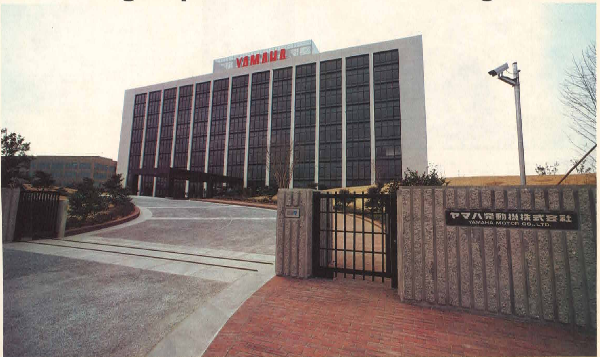
The new R & D Center is a steel-frame 8-storyed building with one underground floor. It is 35.11 meters high and total building area is 23,910.58m 2 . (taken from front entrance side)
