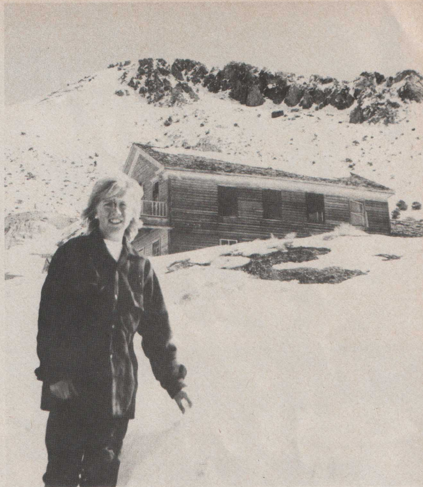
The American Hotel rising behind Larry Lemaster was built at Cerro Gordo in 1871.
