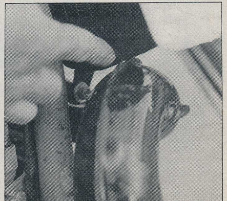
... 'cos if you're not careful the pipe seam will chomp into the base of the rad.
