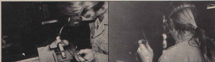
Then clamp each piece tightly and tack-weld seams. Align long seams and weld halves together.
