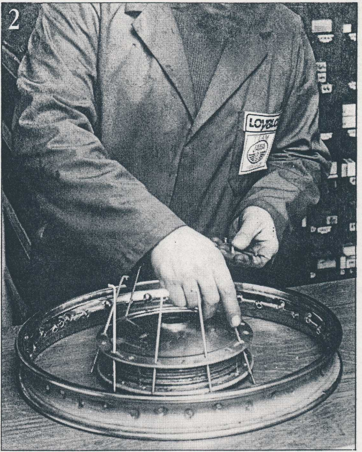
2 A flat surface is all you need to begin with. Insert 'inner' spokes in alternate holes.
