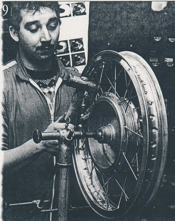
Outer spokes will be curved around the hub unless you gently knock 'em straight.
